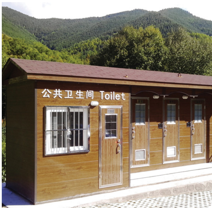
Eco-friendly toilets installed at the top of Wutai Mountain in Shanxi Province. (Landwasher)
